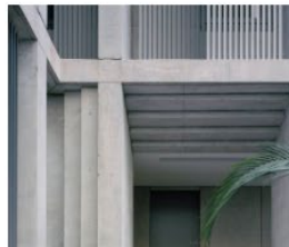
C - OFF FORM CONCRETE PERRY PARK - CANDALEPAS ASSOCIATES
