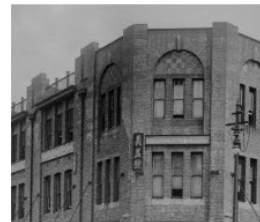
D - EXISTING BRICKWORK 96-100 HAY STREET
